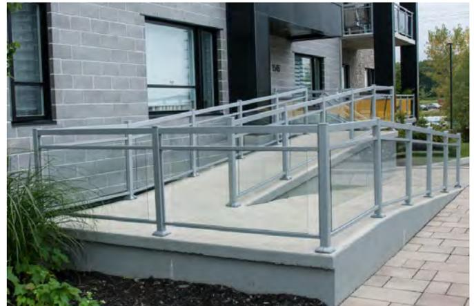
**TABLEAU 1.3 - MAIN COURANTE CONTINUE AVEC VERRE (2 POTEAUX AVEC 1 POTEAU CANNELÉ 1 5/8 x 1 3/4 ENTRE) 0.75 KN/M (BÂTIMENTS COMMUNS)**
